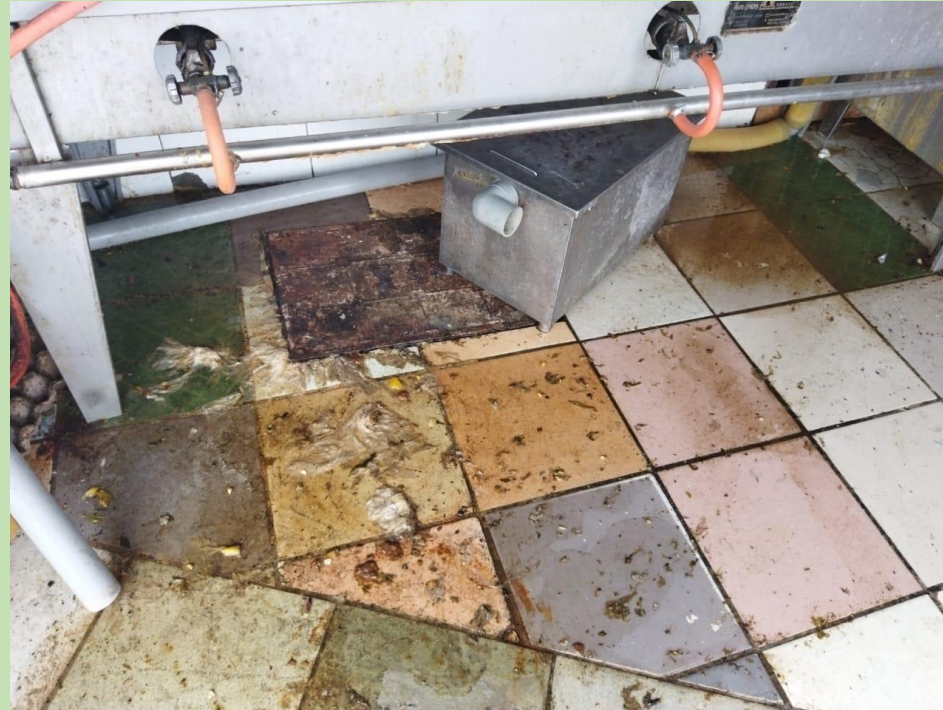
Overflowing septic tanks
